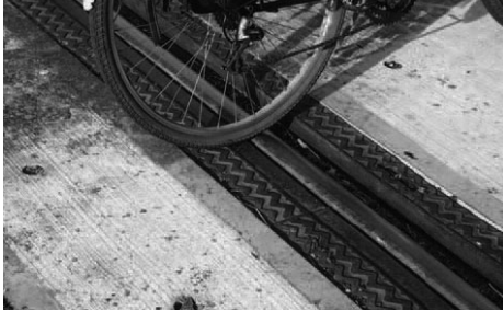
Concrete RR crossing with rubber flanges
