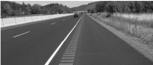
Well placed rumble strip leaves room for bicyclists
